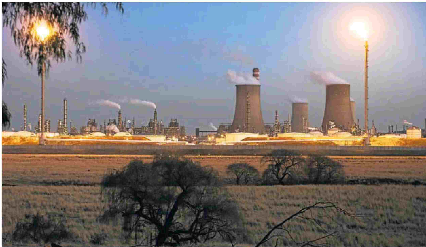
BIGGEST POLLUTER: Sasol in Secunda is the largest synthetic fuels facility in the world, and it produces about 35% of South Africa's liquid fuel needs, including petrol. The plant is also the single largest emitter of carbon dioxide on the planet Picture: GETTY IMAGES
